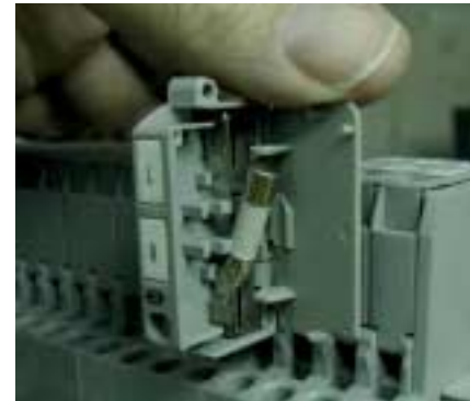
Figure 3-10b, Fuse Replacement
