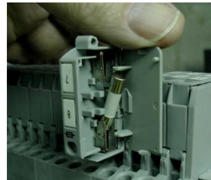
Figure 3-10b, Fuse Replacement
