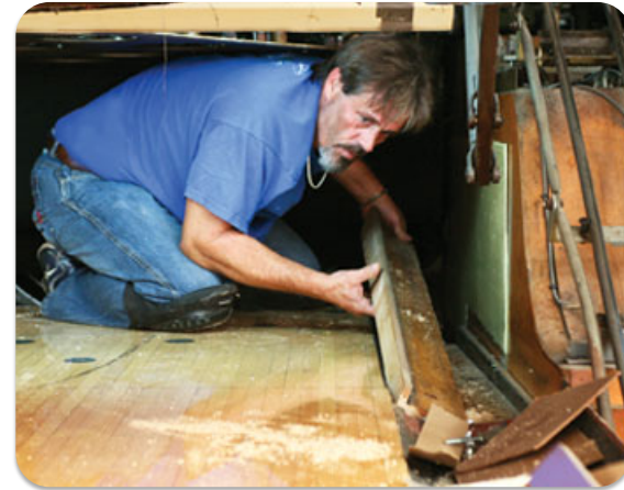
REMOVE PIN DECK AND FLAT GUTTERS
